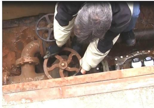
Figure 16 Checking the Inlet Valve
