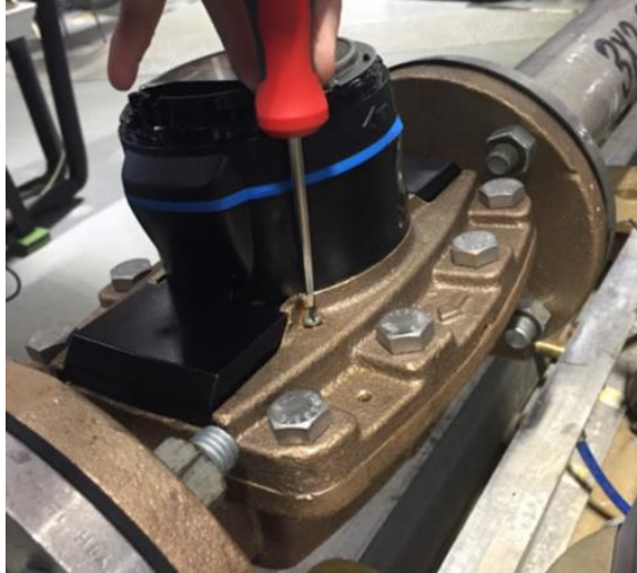
Figure 20 – Turn the Bleed Screw
