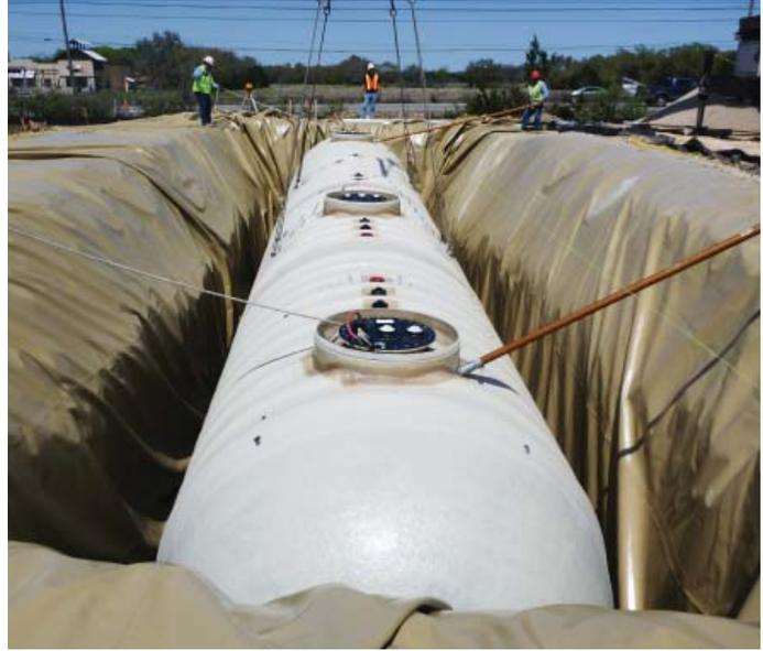
This compartment tank includes 2 bulkheads, an alternative in this limited space to installing 3 individual tanks.
