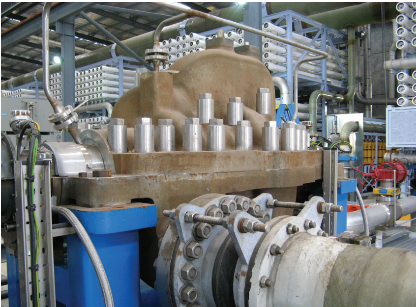
Pump installed at site
